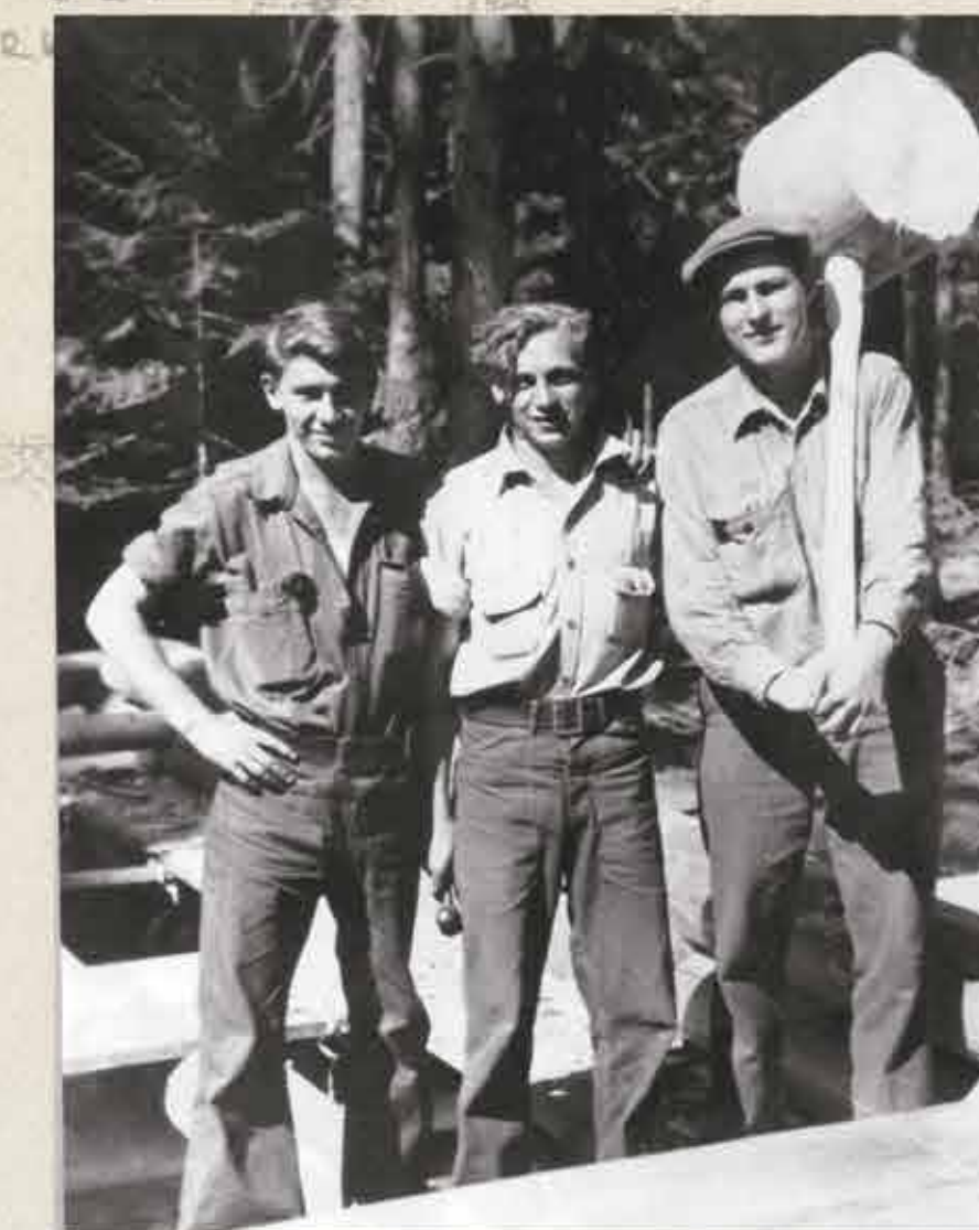
Cecil and James Wylie (left and center) helped build the Luby Bay Cabin
