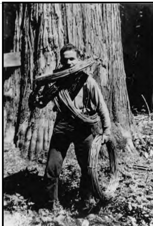
Foreman John Sudneckovich taught recruits how to procure and place the telephone poles and string the lines. With emphasis on safety, he showed the crews how to use and maintain tools and to tighten wires. Improved communication to Priest River and around the lake resulted in a more efficient system for reporting and fighting fires.
