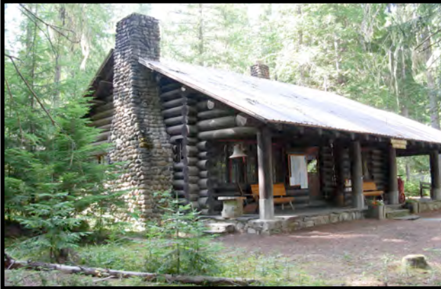
One of the most visible CCC projects remaining is the Priest Lake Museum located at Luby Bay. The rustic log cabin built in 1935-36 housed forest rangers until 1989. Using native materials, CCC crews cut the notched logs, gathered rock for the chimney and fireplace and slate for the front porch. A small CCC mill near Nordman provided the flooring and furniture.
