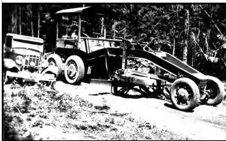
CCC crews assigned to road construction learned to survey roads, dynamite stumps and to drive and maintain equipment. Early roads improved by these crews were Reeder Bay including access and parking at Elkins Resort, Eastside road from Cavanaugh Bay to Indian Creek, Lamb Creek and Squaw Valley. Most area trails were cleared by recruits for access to forest fires or lookouts and signs were added.
